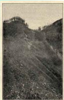
FIG. 13.—PHOTOGRAPH SHOWING HOW ACCUMULATED DIRT IS CLEARED FROM WORKING FACE BY WATER LET IN FROM ABOVE.
